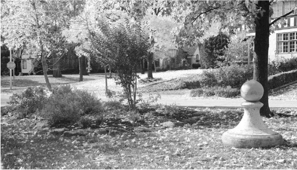
Strawn Park Pedestal After Repair
