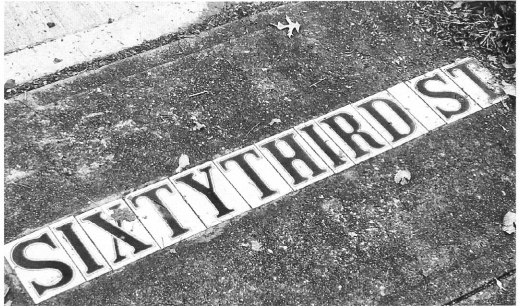
Many street marker tiles are completely missing especially where the City has done storm drain work
